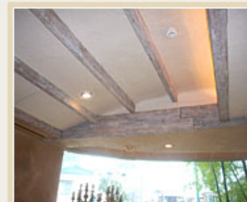
店舗内装・天井見上(3)
